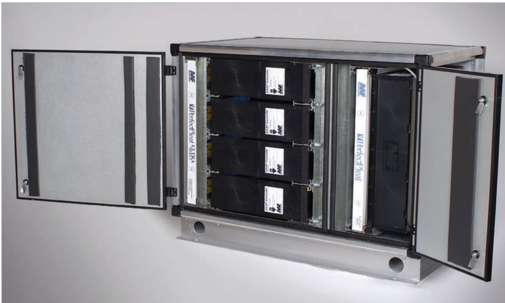
Step 2: The installed high efficiency M-Pak filter.
