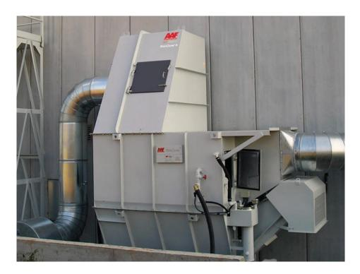
The RotoClone<sup>™</sup> N is a flexible design for a wide range of operating conditions with minimal servicing requirements. Collection efficiencies, including the most challenging particle sizes, are equal to or better than any wet dust collector with comparable energy consumption.
